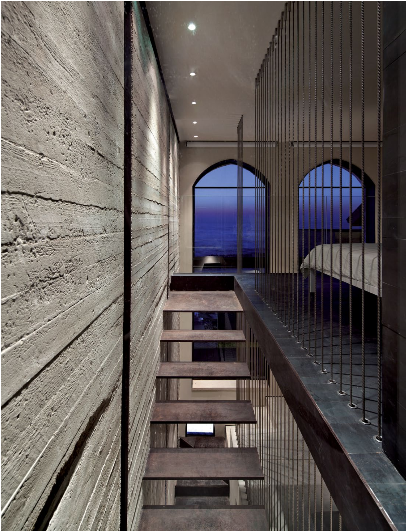
The staircase floats between an exposed concrete wall on one side and a railing of sleek steel cables on the other
